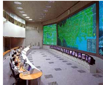
Traffic Control Center
