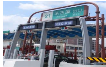
Toll collection system
