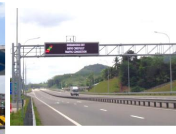
Traffic control system
